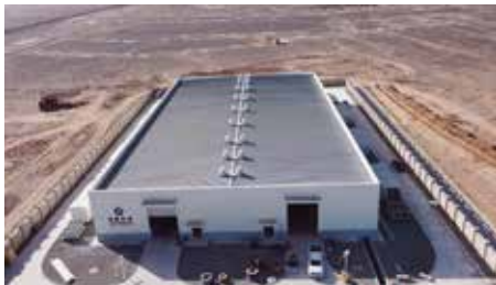
Gansu Guazhou Beidaqiao Baiyang Wind Power Supporting Energy Storage Project
